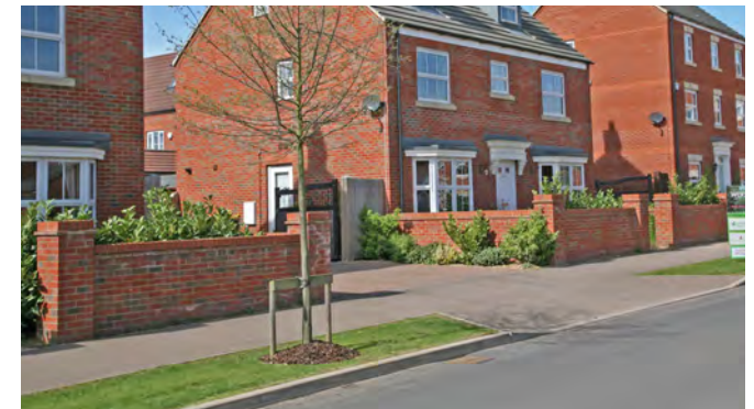
An example of consistent and high quality boundary treatment.
